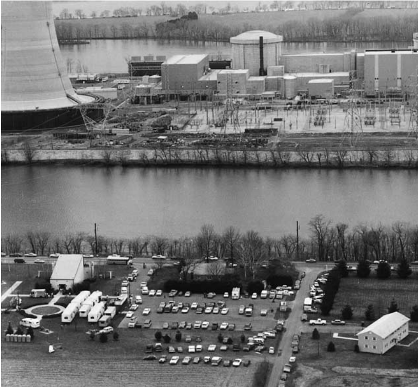
Figure 18. An early stage of Trailer City, looking west. The TMI-2 plant is at top center. The observation center is the white building with the slanted roof. Dewey Schneider's home stands to the right of the observation center among the trees. The cornfield at the bottom of the photo served as a helicopter landing area (National Archives 220-TMI-DE9040025-29).
